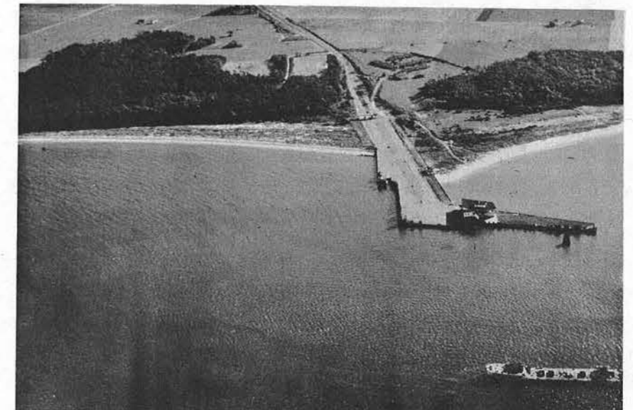
Plate 1 Kiptopeke Ferry Pier
